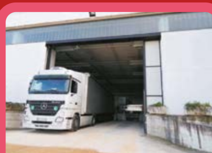
Magazzino carico merci Warehouse load trucks
